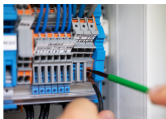
Conductor termination
